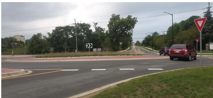
The roundabout installed in 2017 at Nixon Road, Green Road and Dhu Varren Road has improved traffic flow.
